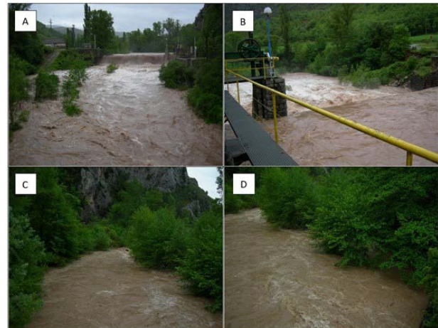
Figure 10. Photographs of the June 2008 flood in the Senterada weir, which affected the sampling area. A: View of the weir from downstream; B: View of the weir from upstream; C and D: View of the trees in the sampling area closest to the channel (Source: Maite Arilla).
