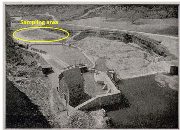
Figure 7. Sampling area on the banks of the Flamisell River indicated in a photograph published in 1922, after the construction of the Senterada-La Pobla de Segur complex (1919-1920). The total absence of riparian vegetation is observed after the construction of the infrastructure (Source: Galí, 1922).
