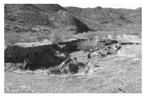
Fig. 2. Gully erosion derived from piping in large-bank terrace.
